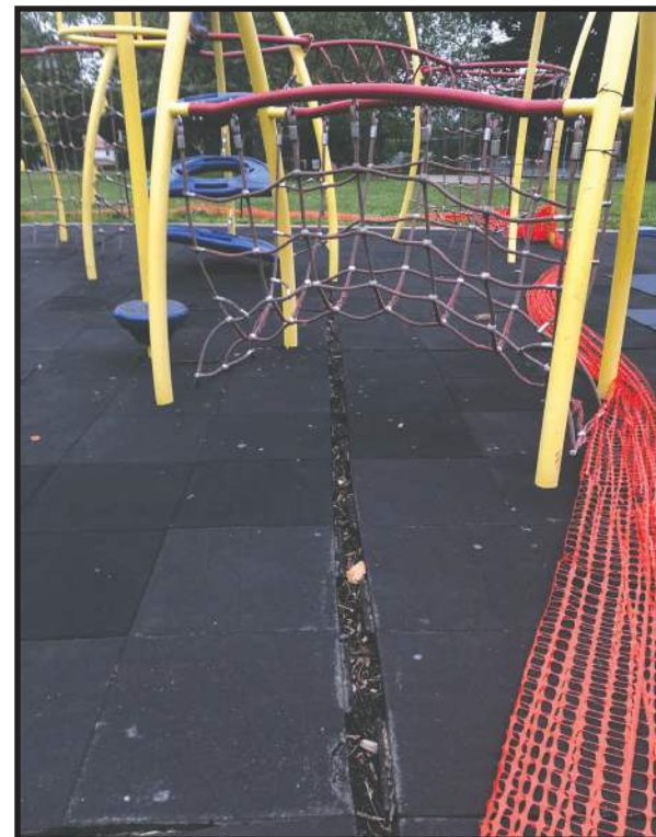
Rubberized surface tiles have separated in several areas, creating tripping hazards.
