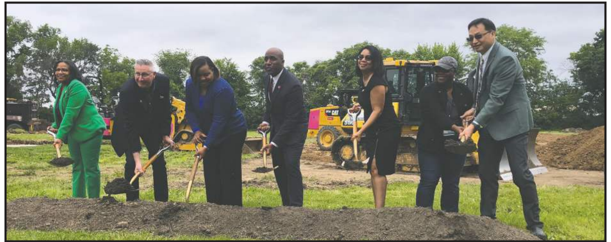
Signaling the start of construction, the May 21 groundbreaking ceremony included Sheron Fulson (PIAC Committee), Parks Director Chris Cotten, Melissa Robinson (City Council Third District), Mayor Quinton Lucas, Melissa Patterson Hazley (Third District-At-Large), project manager Keisha McCoy, and Parks Deputy Director James Wang. Photo by Dorri Partain
