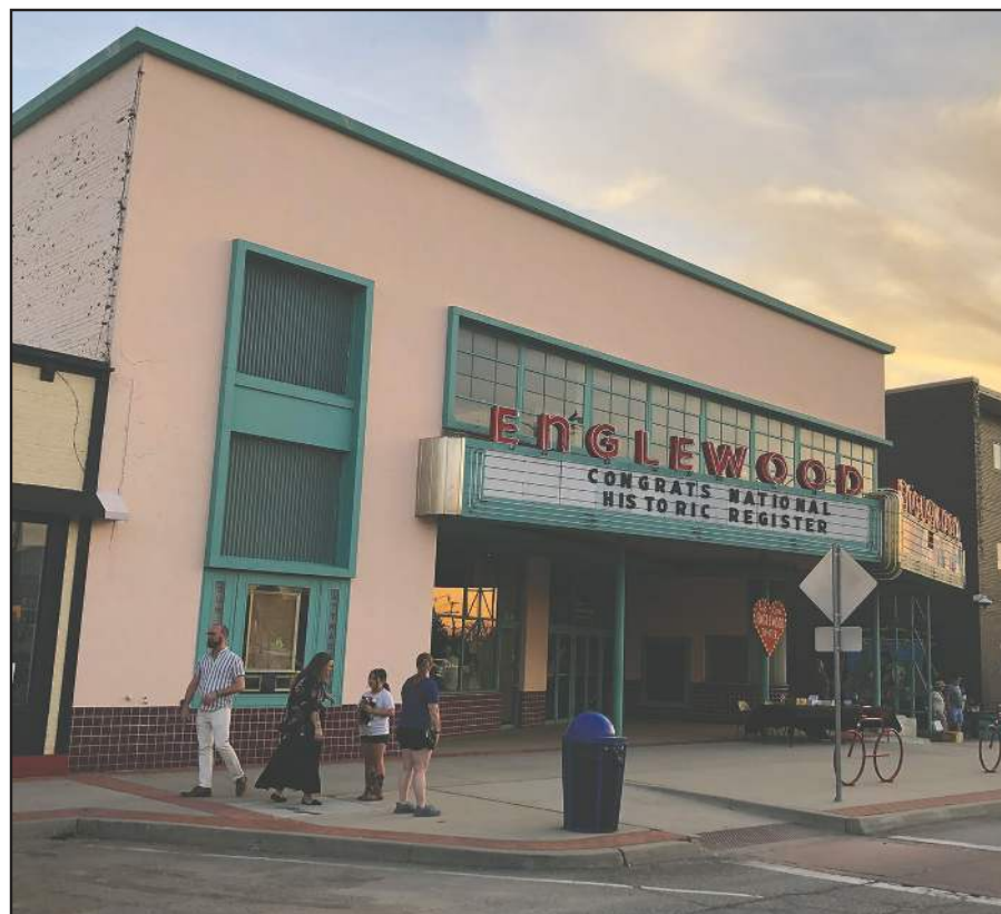
Built in 1949, Englewood Theater has retained its Modern Movement International style and original marquee.
