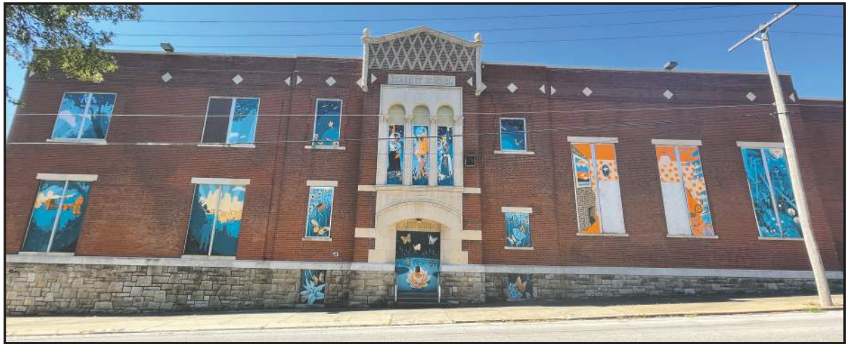
Scarritt School, 3509 Anderson Ave Photo © Northeast News, 2022
