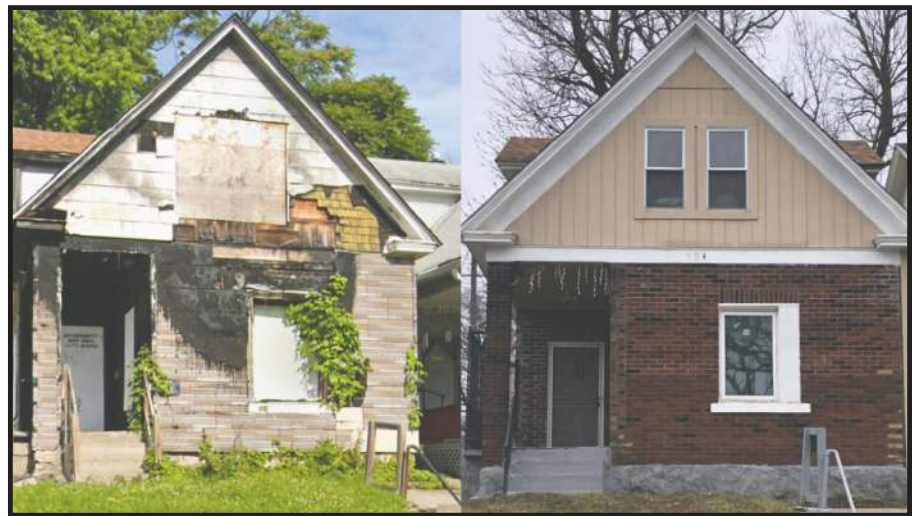
534 Denver Avenue before (left) and after (right) rehabilitation.
