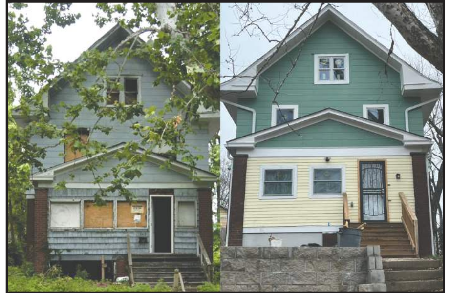
342 N. White Avenue before (left) and during (right) rehabilitation.
