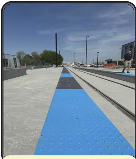
Current Progress of KC Streetcar Riverfront Extension. | Photo by Julia Williams
